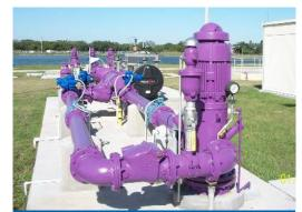
In 2015 Veolia completed a capital upgrade contract at Palmetto for construction management, startup and now O&M services for a new Class V ASR Test Well Pumping and Treatment System, Aquifer Storage and Recovery. The ARS allows the City's treatment plant to inject excess reclaimed water during wet seasons into the ground for storage, which then can be withdrawn to use during higher demand and drier seasons. The work was coordinated by our O&M team at and managed by our regional CPM group.
